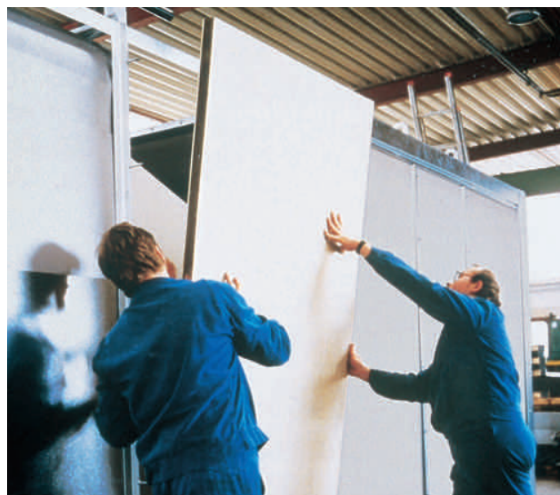
Assembly of PROMATHERM® composite elements to a steel frame construction
