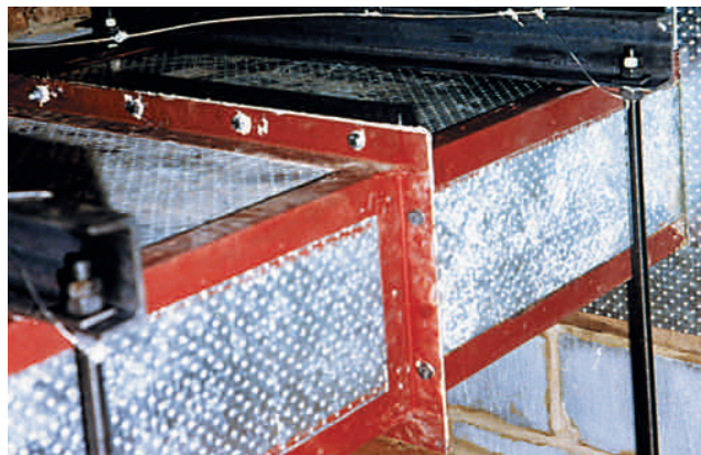
Lining of a duct
